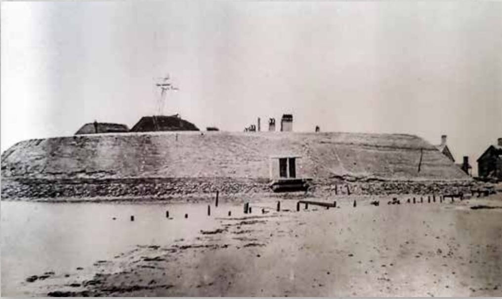
By the end of the war, Castle Pinckney was encased behind tall, sloped earthen sand and sodded walls. This circa 1865 photograph shows the western wall of the fort. (Matthew Locke Collection)
