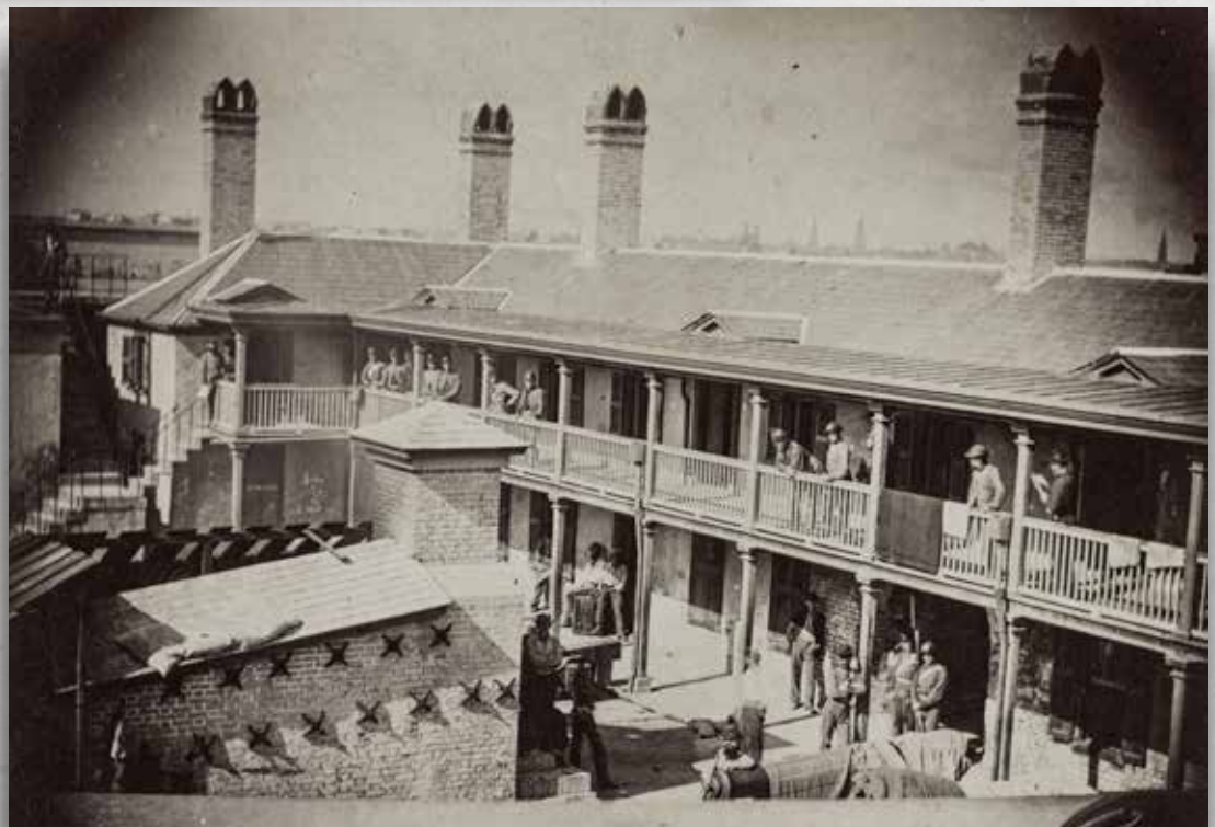
Interior of Castle Pinckney showing the barracks, hot shot furnace, and blankets covering an unmounted smoothbore cannon. The hot shot furnace was converted to an oven during this time. (Library of Congress)
